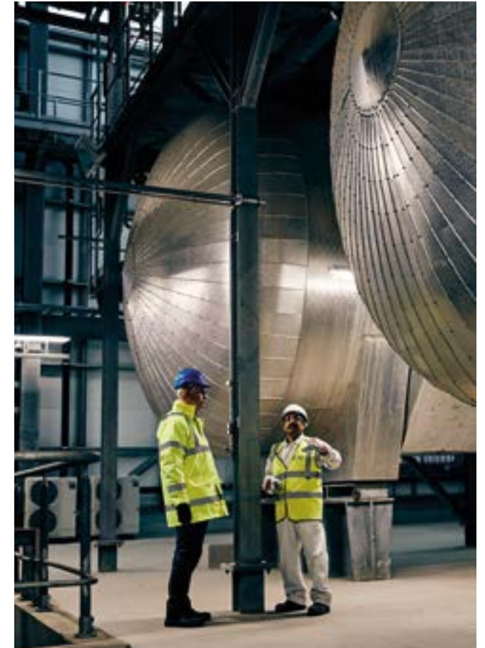
The two feed water tanks at Riverside have a capacity of 150m 3 each and an operating level of 80m 3 .
