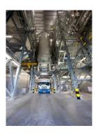
The resultant residue left on the filter bags is termed Air Pollution Control residue (APCr) and this is collected in 3 silos. APCr accounts for approximately 3-4% of the facility's waste throughput and in 2016 the facility recycled approx. 50% of the APCr produced at site. The remainder of the APCr was sent for disposal at a licensed hazardous waste site.
