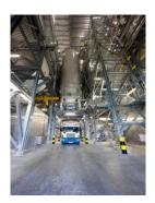
The resultant residue left on the filter bags is termed Air Pollution Control residue (APCr) and this is collected in 3 silos. APCr accounts for approximately 3-4% of the facility's waste throughput and at present and is sent for disposal at a licensed hazardous waste site. In 2014, methods for recycling APCr were trialled and, after proving to be successful, the facility now recycles 40-45% of the APCr produced at site.
